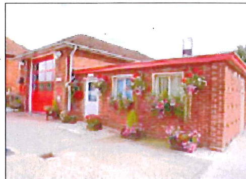
Brinklow Fire station—Heath Lane
